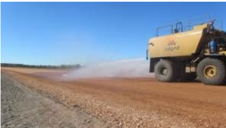
Figure 15 - Water cart dust suppression
